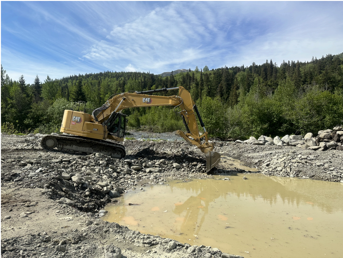
Figure 2. Rewatering a side channel of Resurrection Creek following restoration of the previous mine site. (NOAA)
